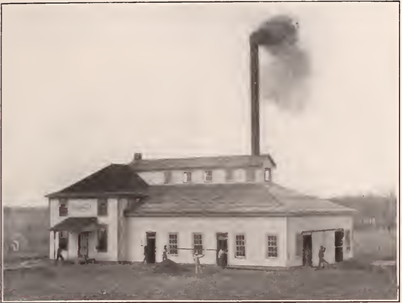
POWER PLANT OF THE OKOLONA SCHOOL, MANNED BY THE STUDENTS
